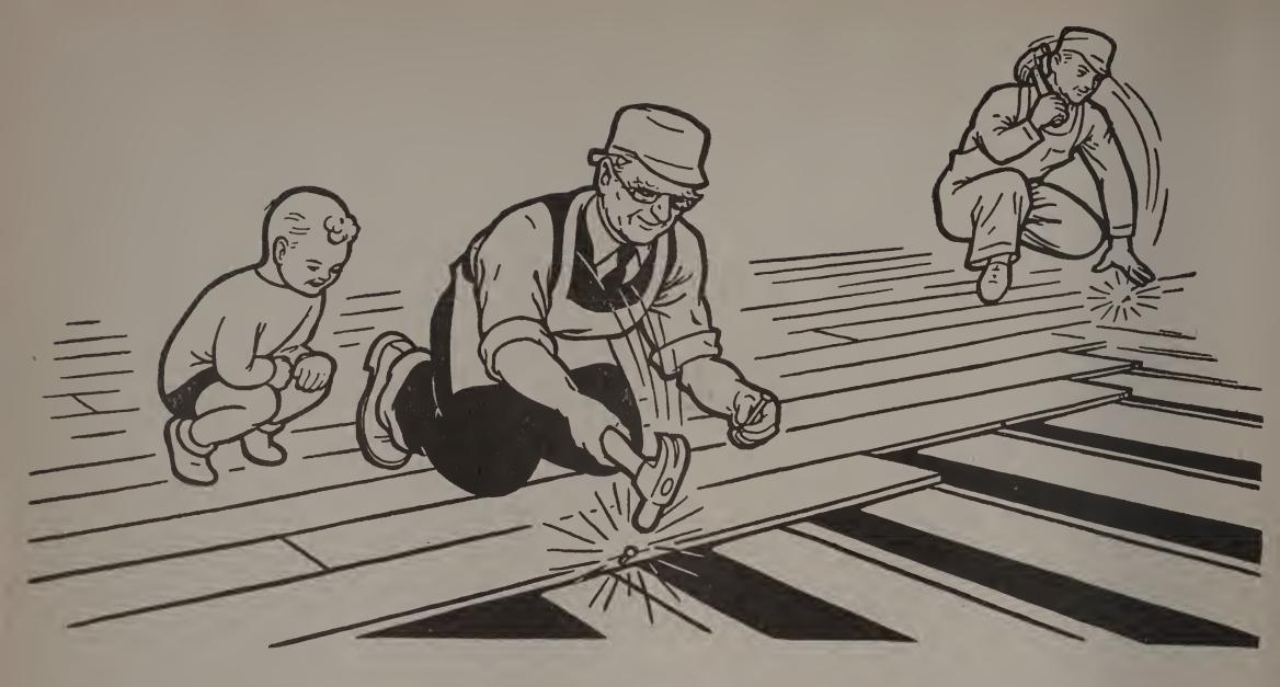
After the joists had all been nailed down, they were covered with wide, thin boards. These made the floor. Each board was fitted tightly to the board next to it. There must not be any cracks in the floor! Little Chips watched Chips and his helper as they fastened the floor boards with nails. It looked very easy to him.
